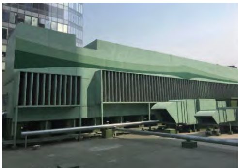
(a) 冷却塔隔声罩
